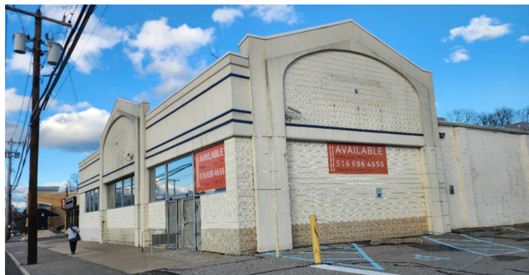
South Facing View
